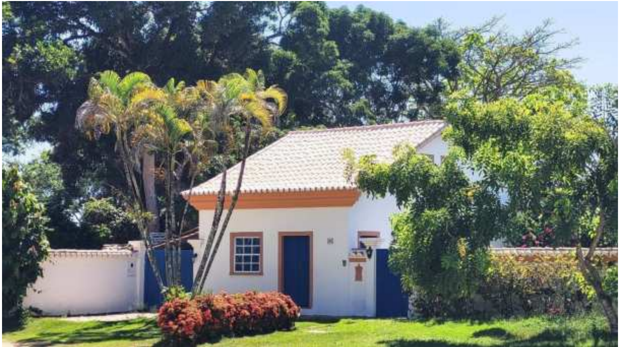
House in the upper town
